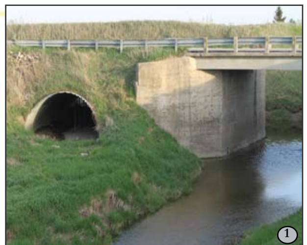
1. Wildlife culvert systems like this one can have a large impact on reducing road mortality.
