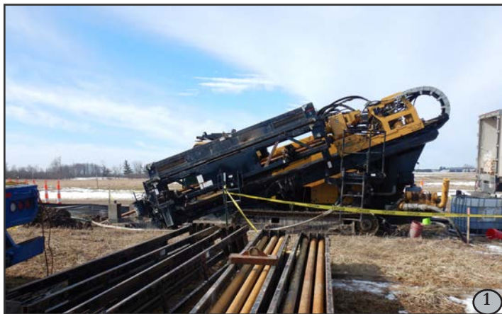
1. HDD machinery and workspace.
