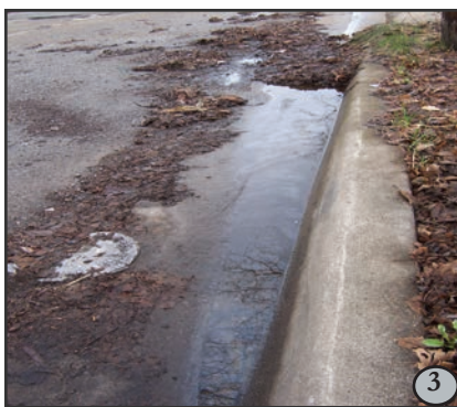
3. Storm water runoff carries road salt, pollutants from vehicles, and warm water into storm sewers, some of which lead directly to rivers and other water bodies.
