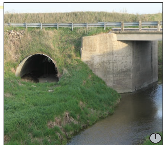
1. Wildlife culvert systems like this one can have a large impact on reducing road mortality.
